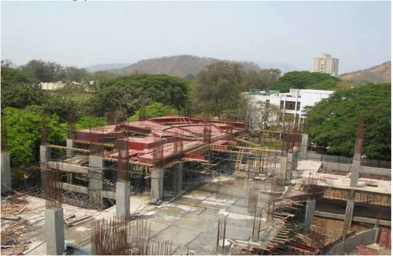
Actual Work Photograph taken on March 31, 2008
