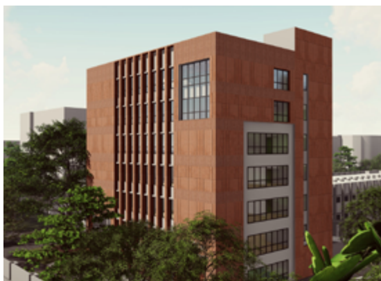
Humanities & Social Sciences (HSS) Annex Building
